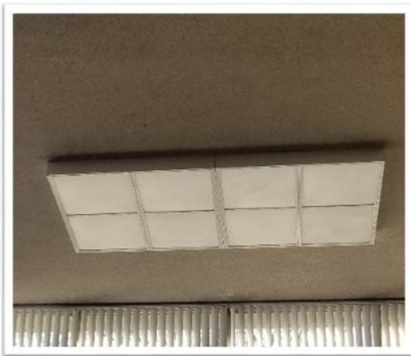
HIGH CEILING AREA
